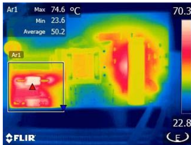
Figure 12 – 90 VAC, Full Load. Ambient = 22.8 °C. Transformer = 65.7 °C. Rectifier Diode = 74.6 °C.
